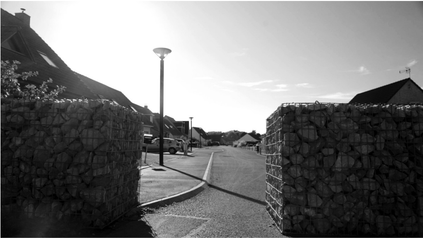
Figure 3.2 The gabion wall blocking vehicle access to Konin I district in Hénin-Beaumont.
